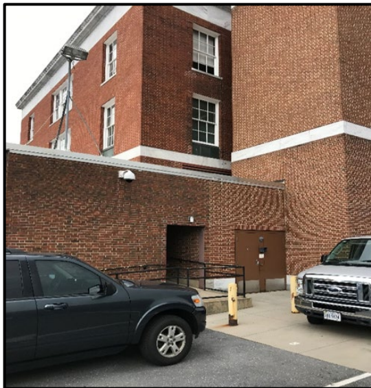
Harrisburg, PA - Prisoner delivery area. No enclosed vehicle sallyport. A new U.S. Courthouse is currently under construction.
