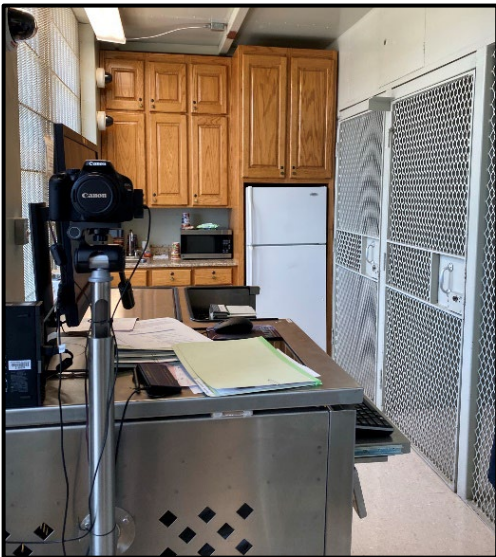
Alexandria, LA – Combined area with holding cells, kitchenette, and prisoner processing. Should be located separately.
