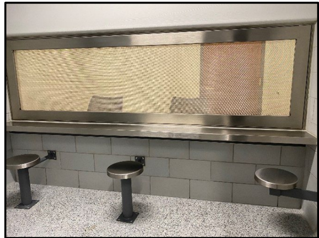
Greenville, SC (New U.S. Courthouse) – Prisoner side of a multi-defendant interview room (completed July 2021).
