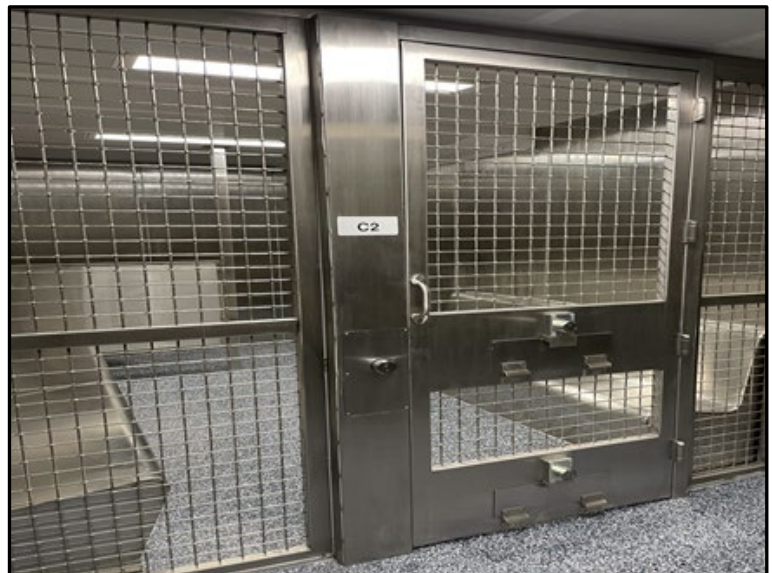
Marquette, MI – Renovation completed June 2021.
