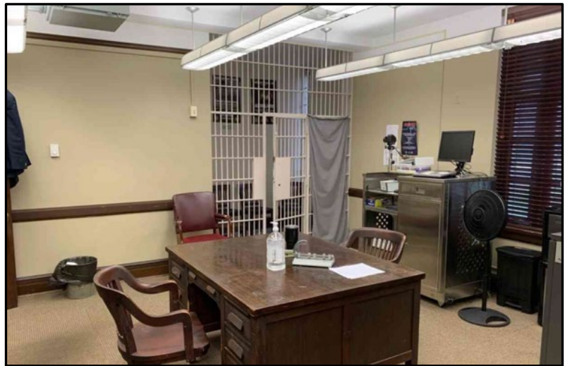
El Dorado, AR (planned renovation) – Antiquated USMS office dating to 1900s. Holding cell, prisoner processing, and Deputy U.S. Marshals space in one area. Each should be located separately.
