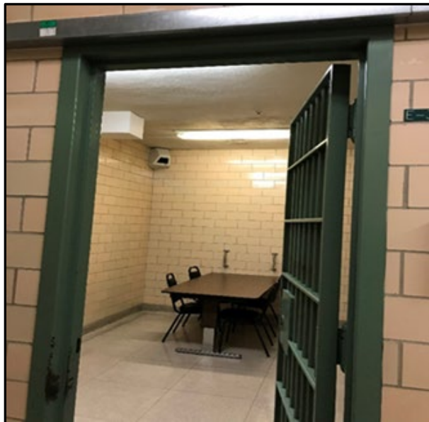
Washington, DC – District Court interview room. No prisoner/attorney separation, plaster ceilings, antiquated door does not provide sight/sound separation.
