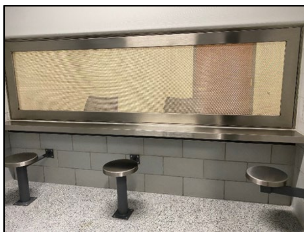
Greenville, SC New U.S. Courthouse – Prisoner side of a multi-defendant interview room (completed July 2021).
