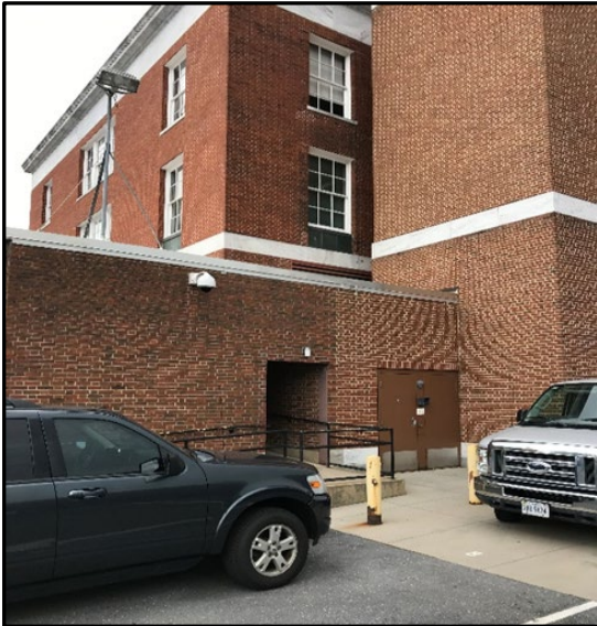
Harrisburg, PA – Prisoner delivery area – the vehicle sallyport is not enclosed. A new U.S. Courthouse is currently under construction.
