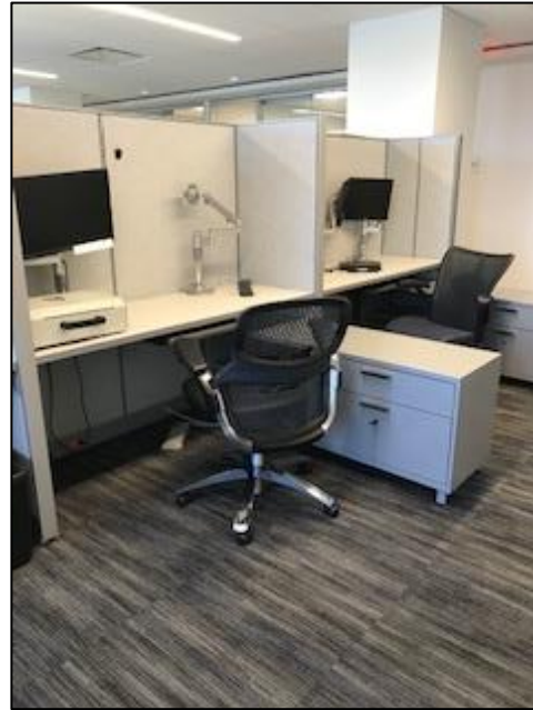
Arlington, VA: New, more durable carpet; squares allow for isolated replacement.
