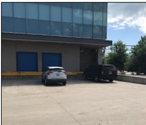
Pierre, SD: Prisoner unloading outside directly next to public sidewalk and main street. No secure prisoner vehicle sallyport.
