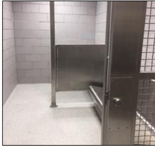
Durango, CO: Newly renovated detention cell.
