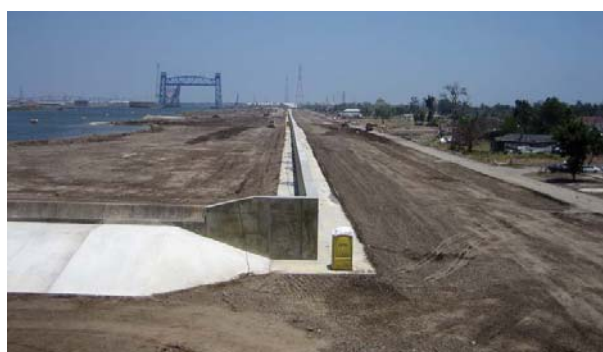
New Floodwall in the Ninth Ward Along the Industrial Canal
