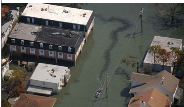
Flooding During Hurricane Katrina (August 2005)
