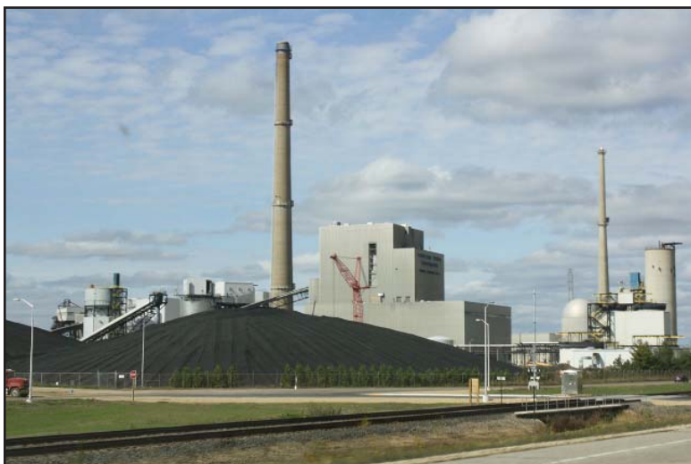
Dairyland Power Cooperative near Genoa, Wisconsin Photo Courtesy of Royalbroil
