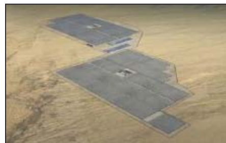
Genesis Solar Energy Project BLM Image
