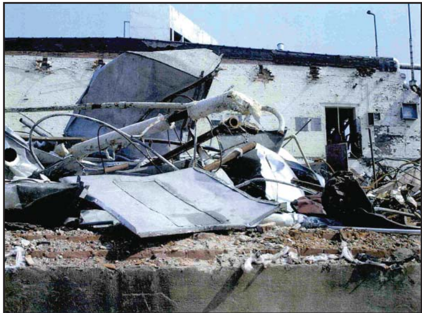
Demolition of Asbestos-Laden Factory in Chattanooga, Tennessee
